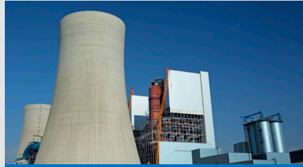
PULVERISED FUEL BOILERS
